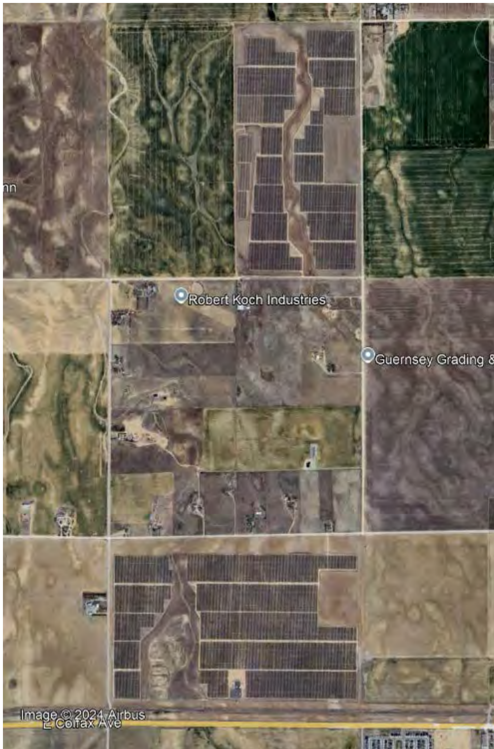
This project was built in 2021 for an 80 MW facility. The closest adjoining home is 270 feet from the nearest solar panel.
